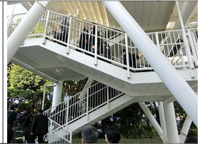
We climbed the Tsunami Evacuation Tower
